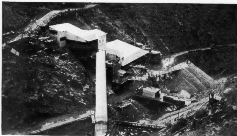
THREE HUNDRED TON flotation mill of the Arizona Molybdenum Corporation in Copper Creek, Arizona. The ore treated contains copper and molybdenum and a 95 per cent concentrate is made
